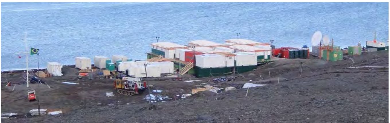
Antarctic Emergency Modules at the site of the Comandante Ferraz Antarctic Station, Admiralty Bay, King George Island, installed in the summer of 2012/2013. Source: SECIRM.
